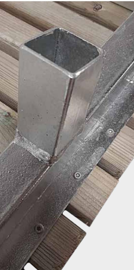
All frames are made of 40x40x2mm square steel tubes, and the connecting legs of 40x40x3mm tubes.
